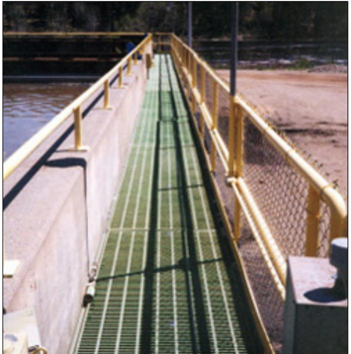
Fibergrate products are engineered to perform in the harshest of environments and need little more maintenance than a washdown. They are durable and can withstand impacts and moisture which would normally destroy standard metal or wood products.
