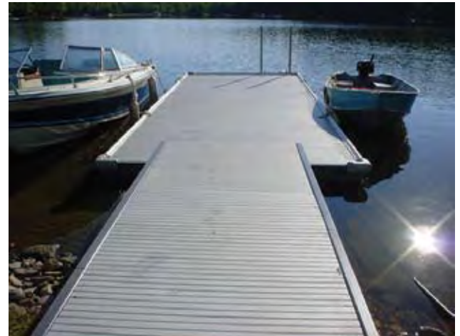
Boat Dock on Horseshoe Lake in Haliburton, Ontario. Safe-T-Span Pultruded Aqua Grate Pedestrian Grating
