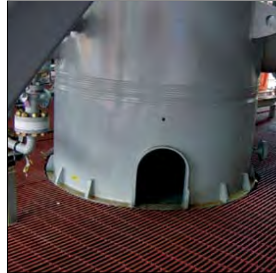
Phenolic pultruded industrial grating used on an offshore platform.
