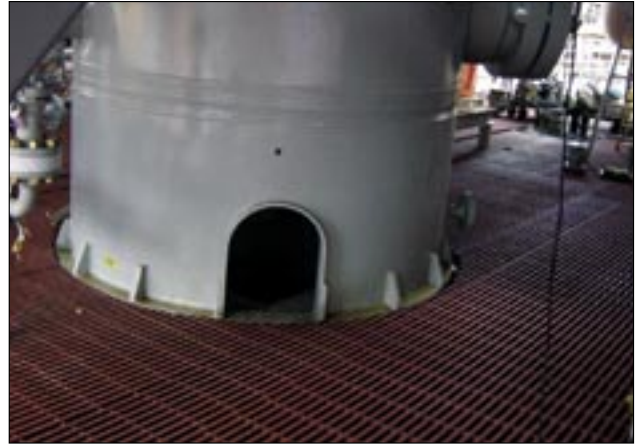
Phenolic pultruded industrial grating used on an offshore platform.
